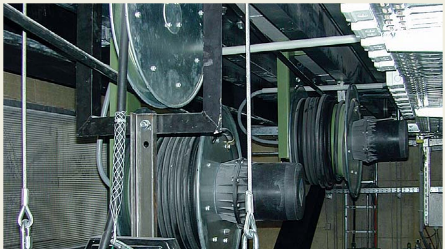
Cavotec Alfo spring driven reels are a common sight in theatre applications around the world.
